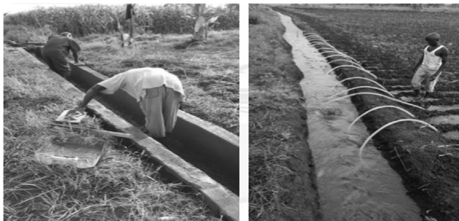
Fig. 3. Improved tertiary and field canals Adopted from Charles (2018).
