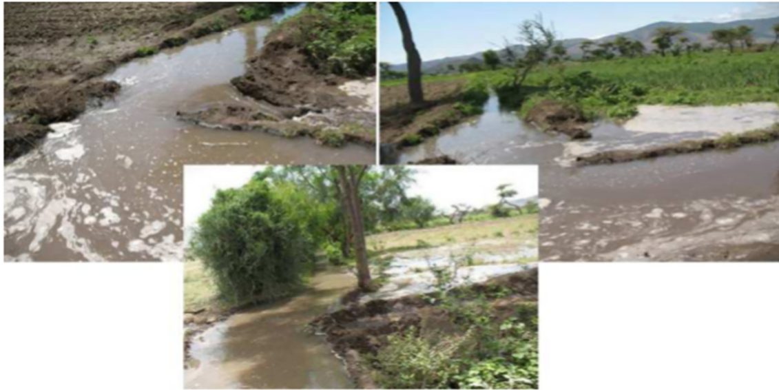
Fig. 2. Overtopping of the main canal at Haleku Melka-Tesso Irrigation project adopted from Lencha (2008) .
